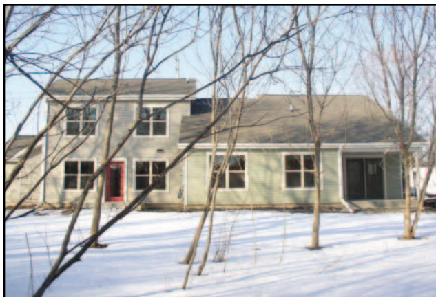
Photo courtesy of NAHB
